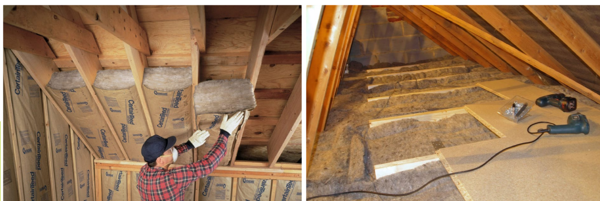
Figure 32 - Different ways to install insulation in attic, in roof (left) and floor (right)
