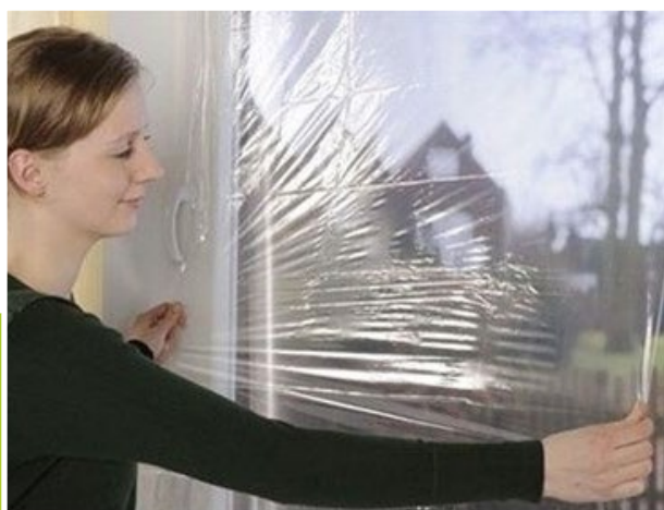
Figure 11 - Installing secondary-glazing film
