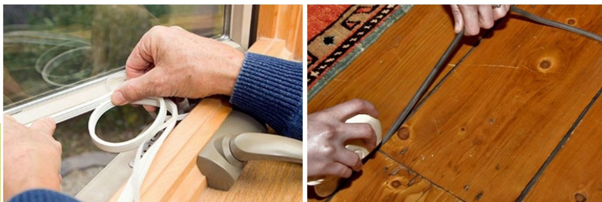
Figure 10 - Draught-proofing windows and floors
