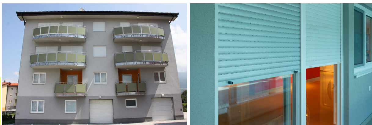
Figure 41 - Roller shutters installed in small residential building
