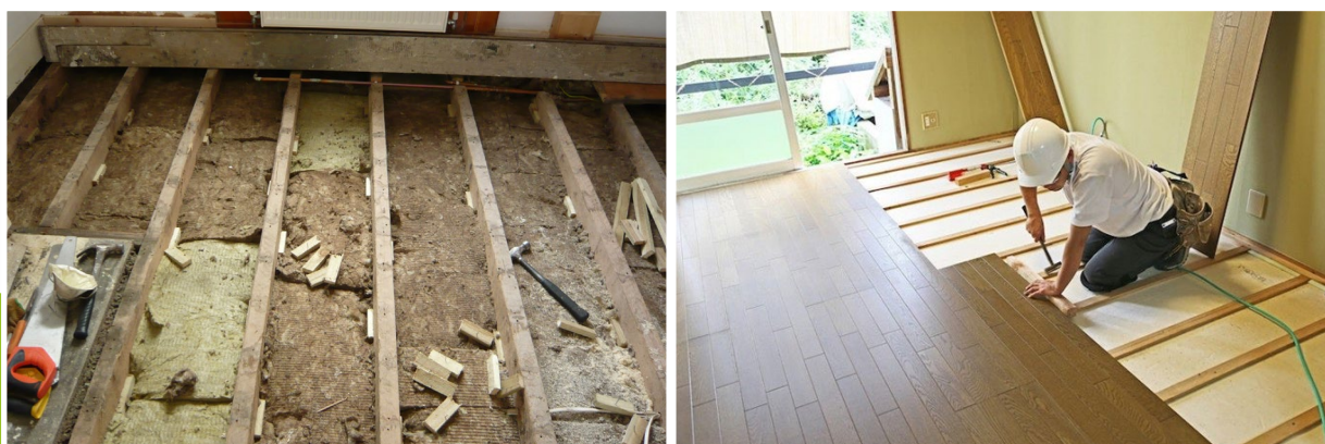
Figure 33 - Examples of installation of thermal insulation of floors
